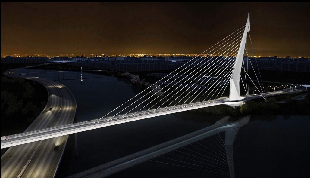
The cable-stayed bridge "The Bridge of Knowledge", built to give research centers in universities access to highways of the city of Rio de Janeiro.
